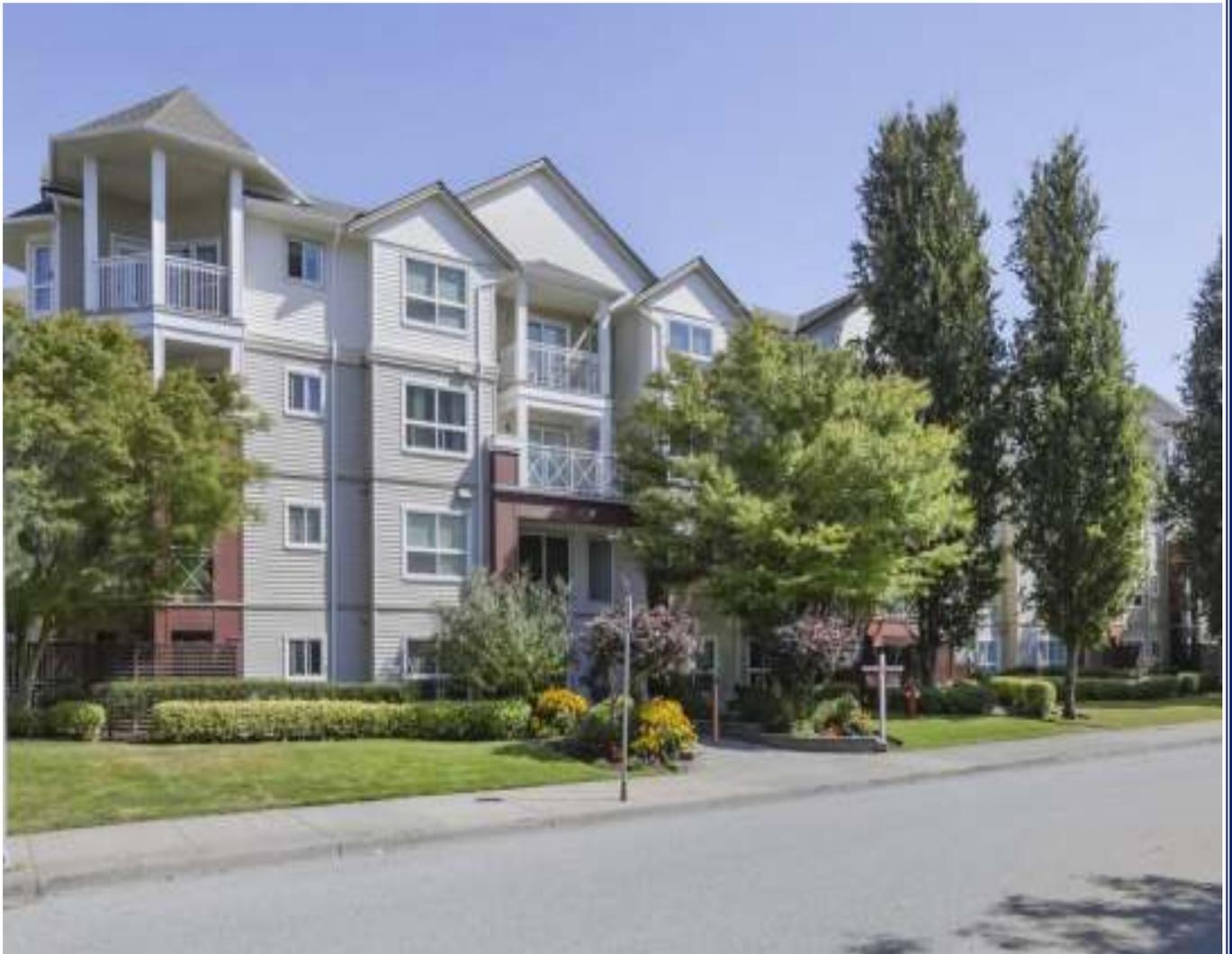
.17) **Montecito By The Sea, White, BC** - Full building envelope restoration project consisting of 3storey (42) units residential condominium building. Existing cladding was replaced with rainscreen fibre cement cladding system. Existing deck membranes, railings, windows, doors and roofs were replaced with new. Conrad Desrosiers, P.Eng. FEC, BEP, RRO, acted as engineer of record on this project while working with other firm.
